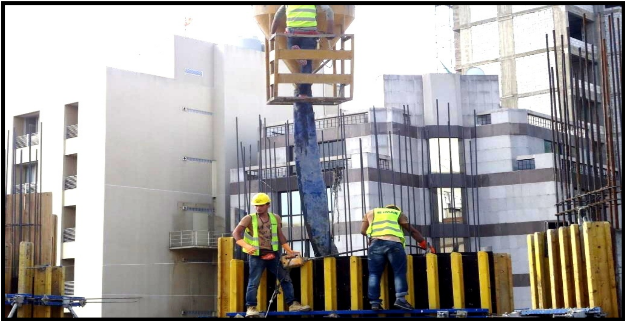
Pouring Of Vertical Elements 3 rd Floor
