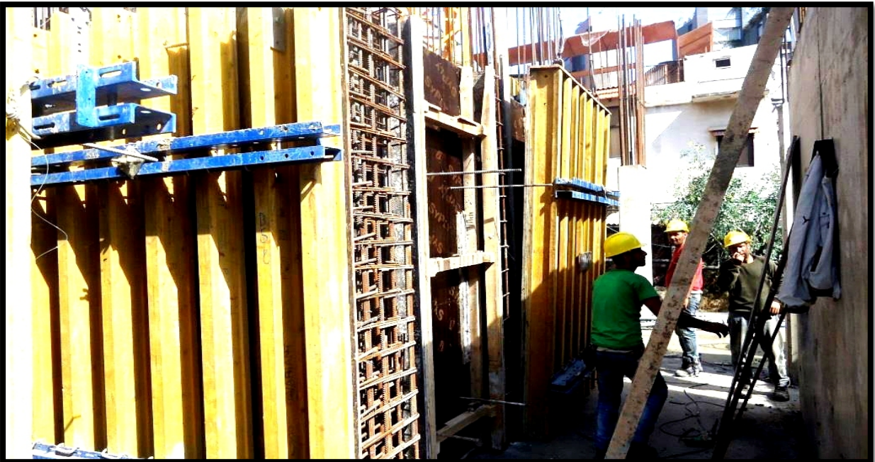
Shuttering Closing Core Wall
