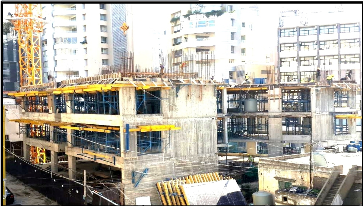
Rebar Works For Vertical Elements 3 rd Floor
