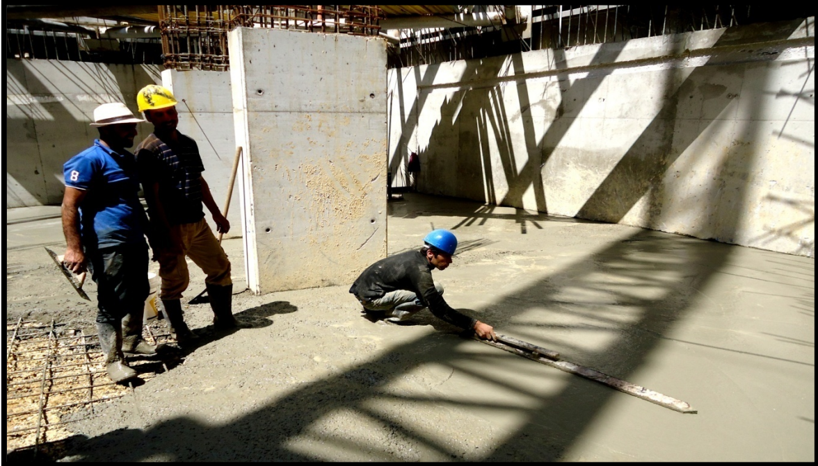
Slab On Grade Casting
