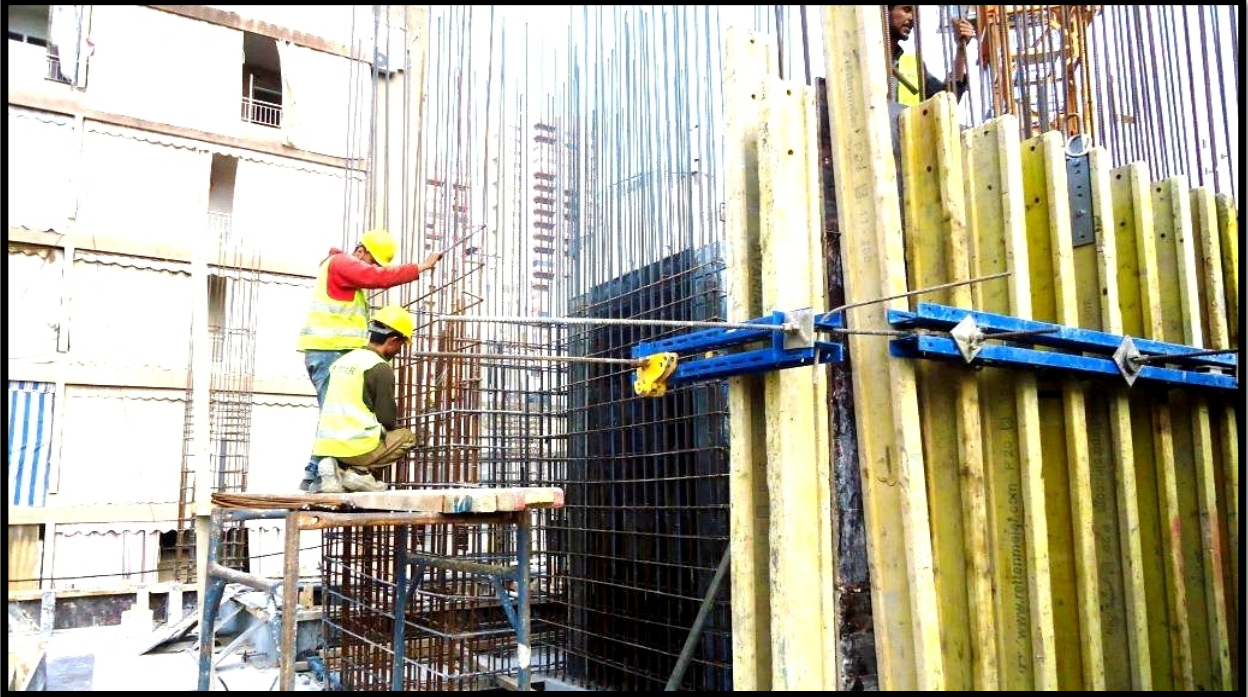
Rebar and Shuttering Core Wall
